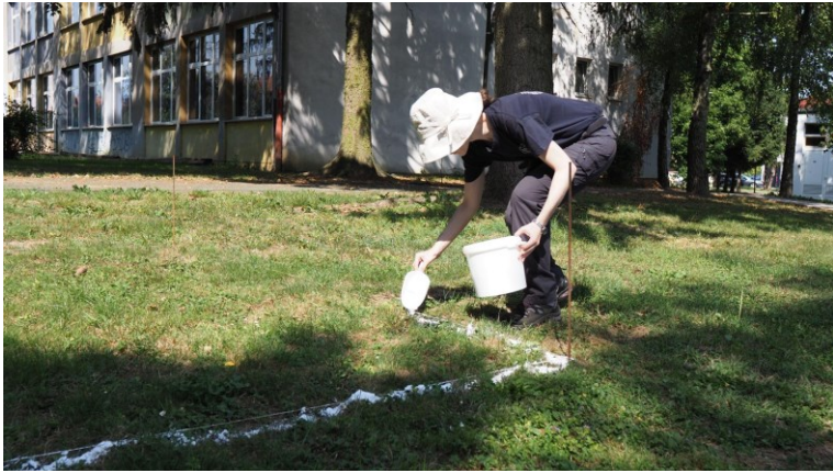
Photos of S2 during the delineation and the excavation of the first layer
